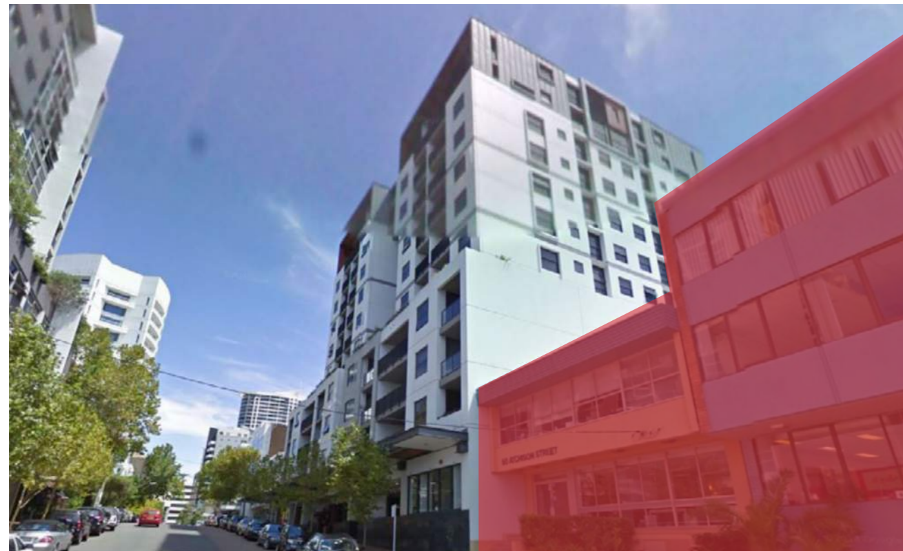
6. SIDE WALL OF ADJOINING RESIDENTIAL BUILDING AT 40-48 ATCHISON STREET
